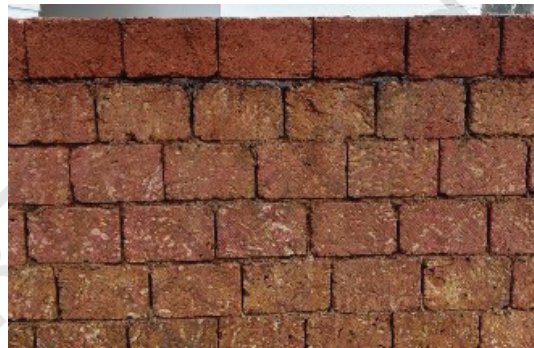
Fig. 11.7: Laterite rocks used as bricks
