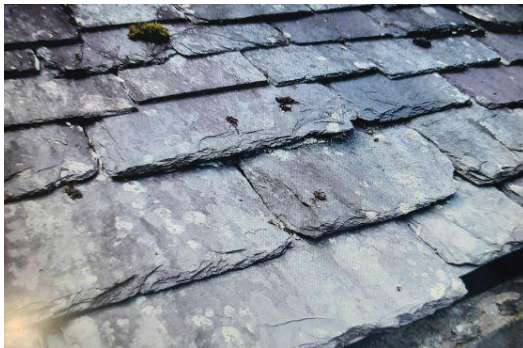
Fig. 11.6: Rocks used for roofing
