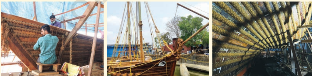
Fig. 7.9. Re-creation of a 5th-century stitched ship
